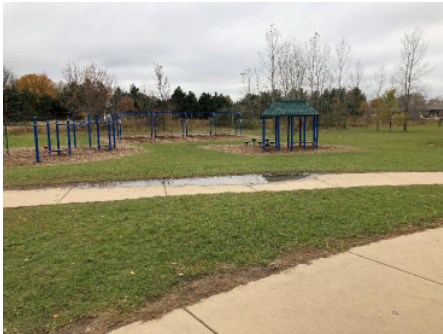
Standing water on new pavement. Additional storm sewer and/or regrading required.
