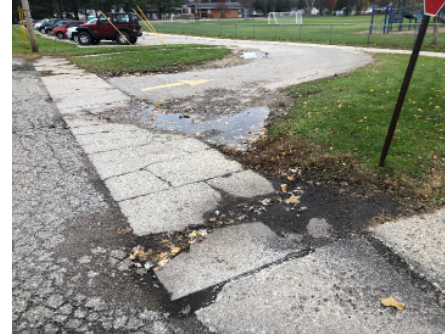
East side of building:
