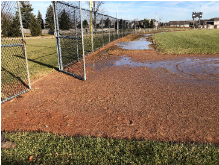
Minor drainage issues at softball field.
