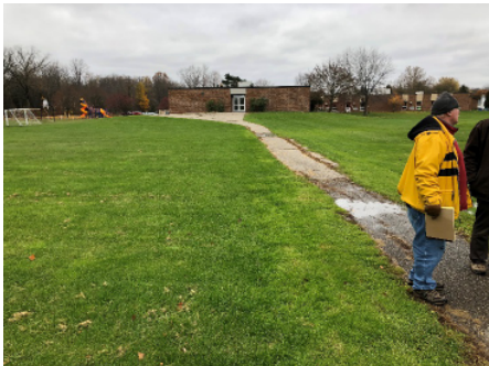
East side of building:
