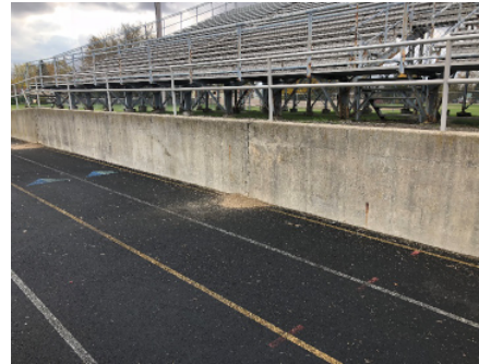
Sinkhole caused by failing storm structure.
