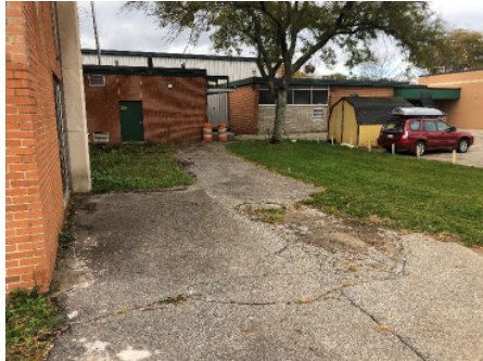
North side of building:
